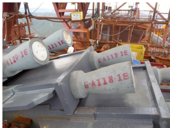
Figure 8. Tower Saddle. Side Span Strand Anchorage
