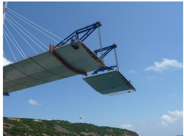
Figure 12. Lifting of Boxes by Derrick Crane
