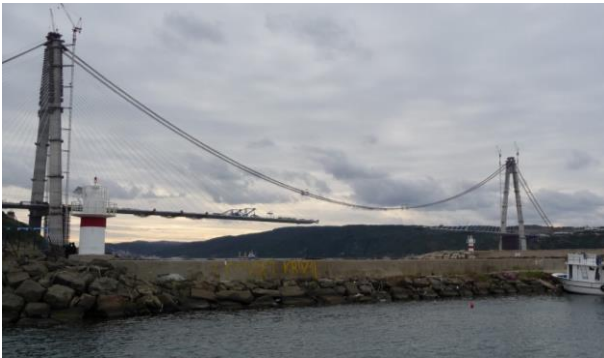
Figure 14. Bridge Deck Erection from Suspension Cables
